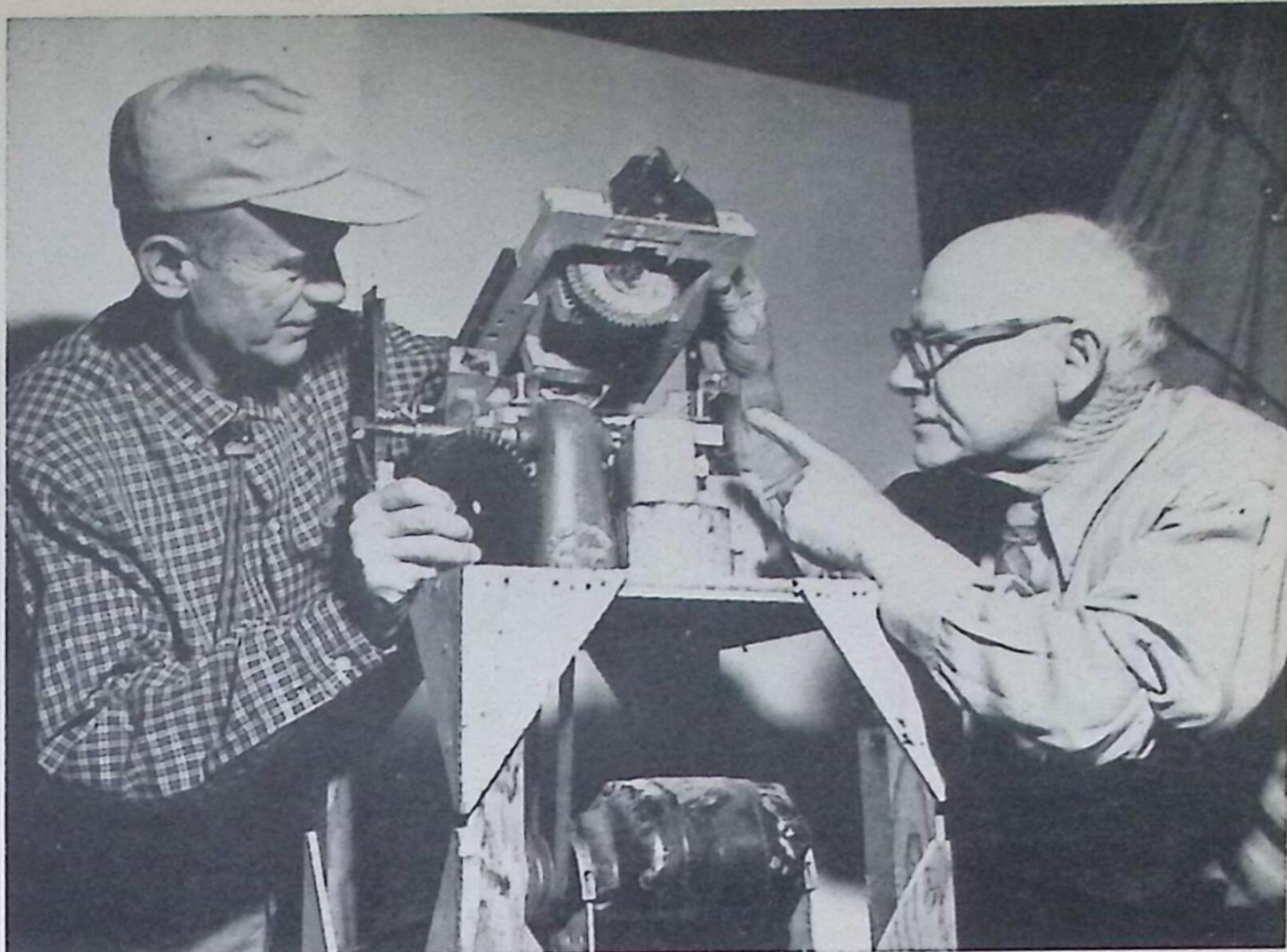
Ted Bhend and Henry Reinecke using special gear cutting jigs devised by Bhend.
